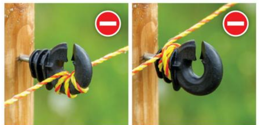
Do not wind the wire on the insulator!
